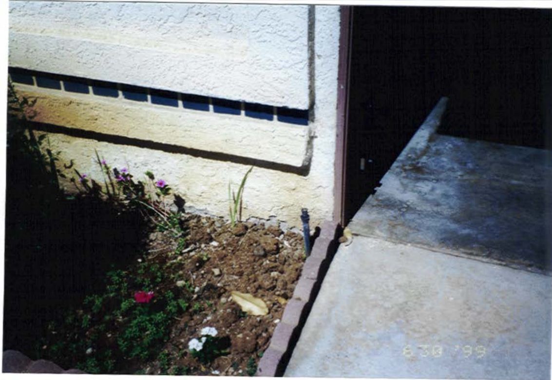
Front yard sprinklers and their proximity to the residence
