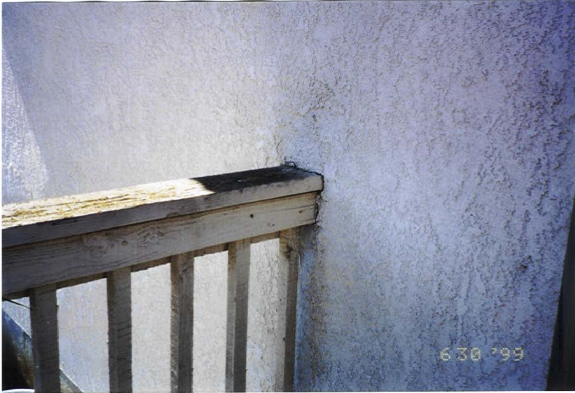
Balcony railing connection (end of roll #2)
