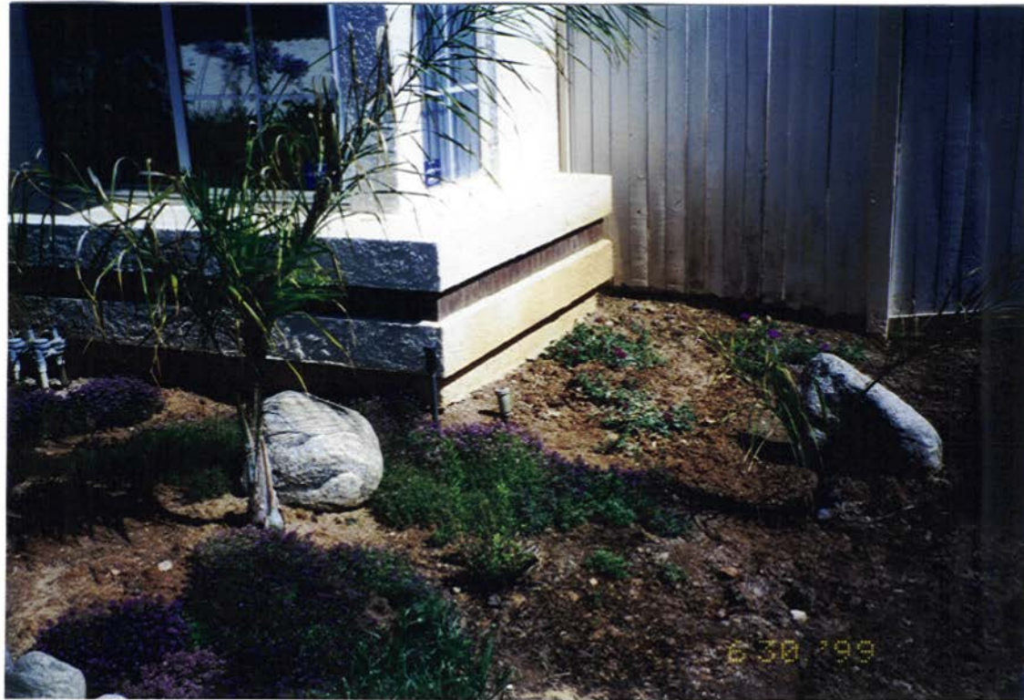
Front yard sprinklers and their proximity to the residence
