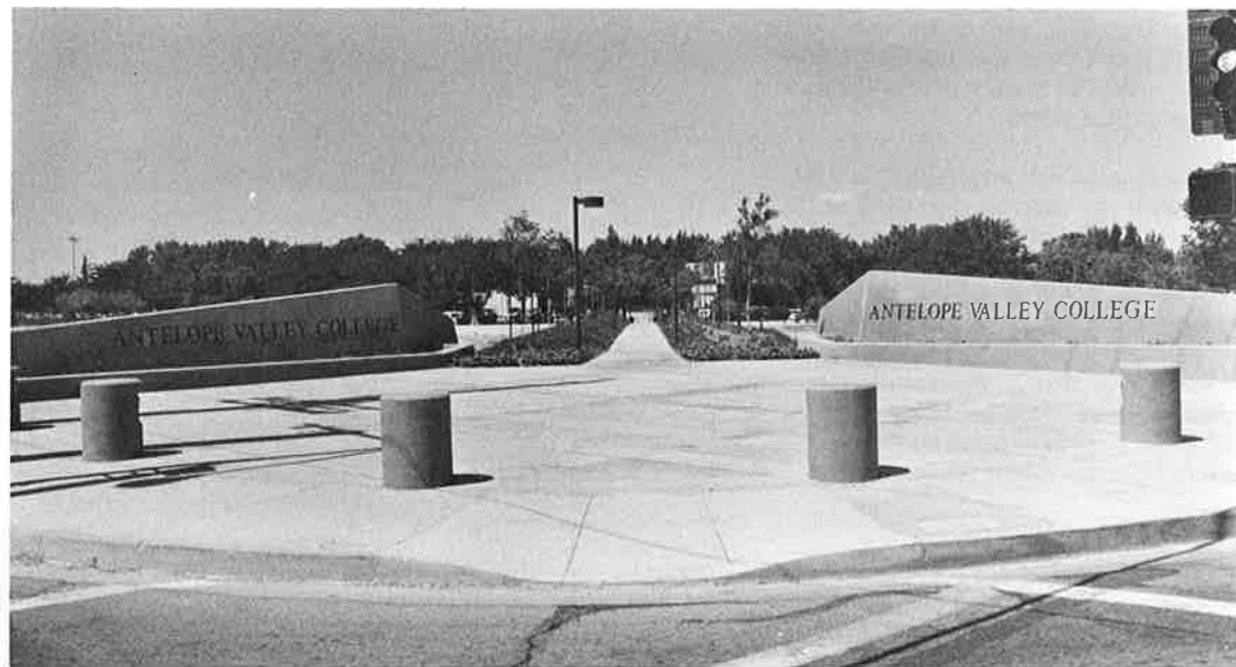
New Main Entry Monument Plaza ---Gives the College a much-needed identity and creates a forecourt to the future Administration building.
