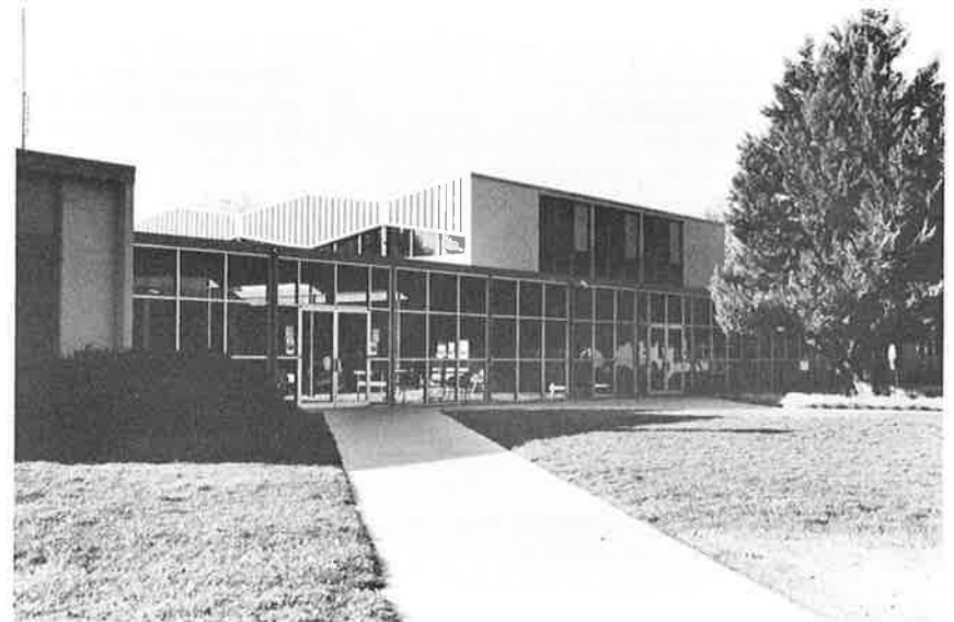
Student Center --- Attractive floated steel roof design with covered walk in foreground which was later glass enclosed due to windy weather
