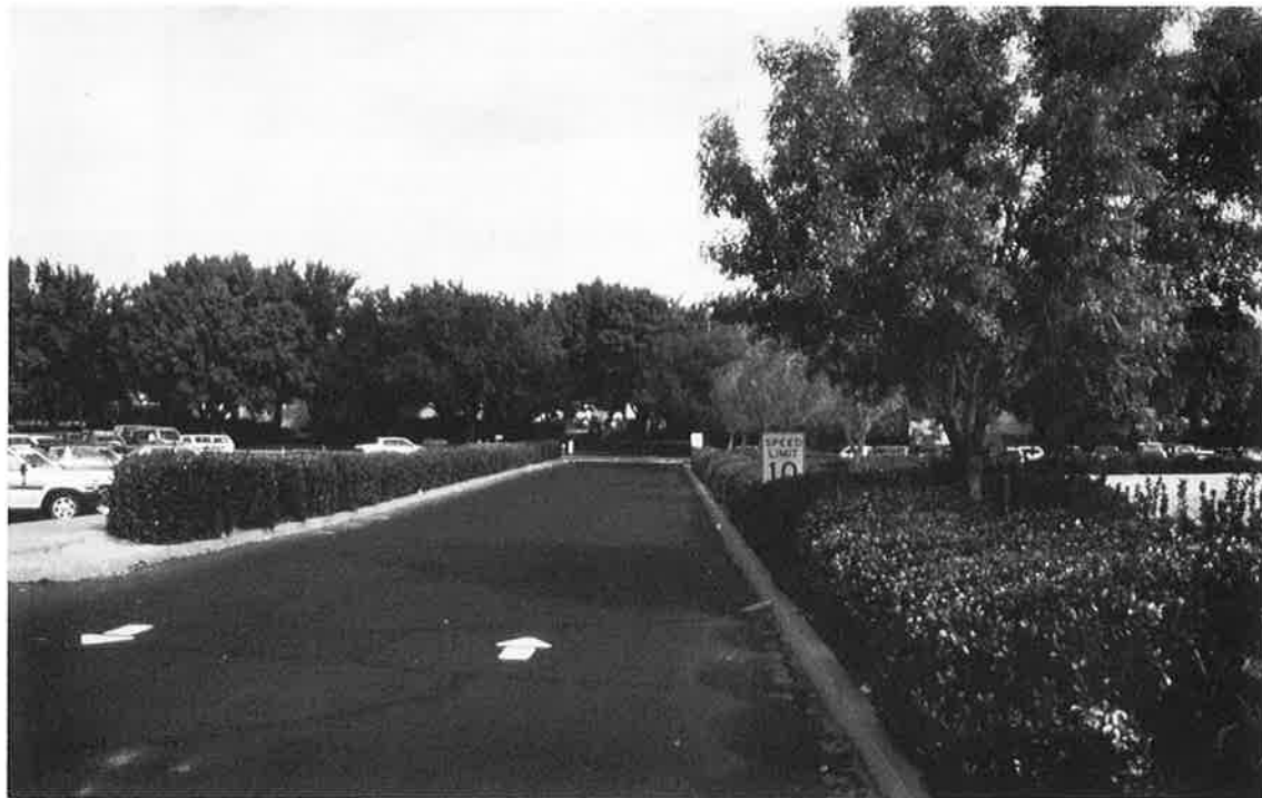
Main Entrance Driveway ---Much too narrow. Recommended to be widened by creating a second driveway and a planted median for a future guard 'shack' or gate, if needed
