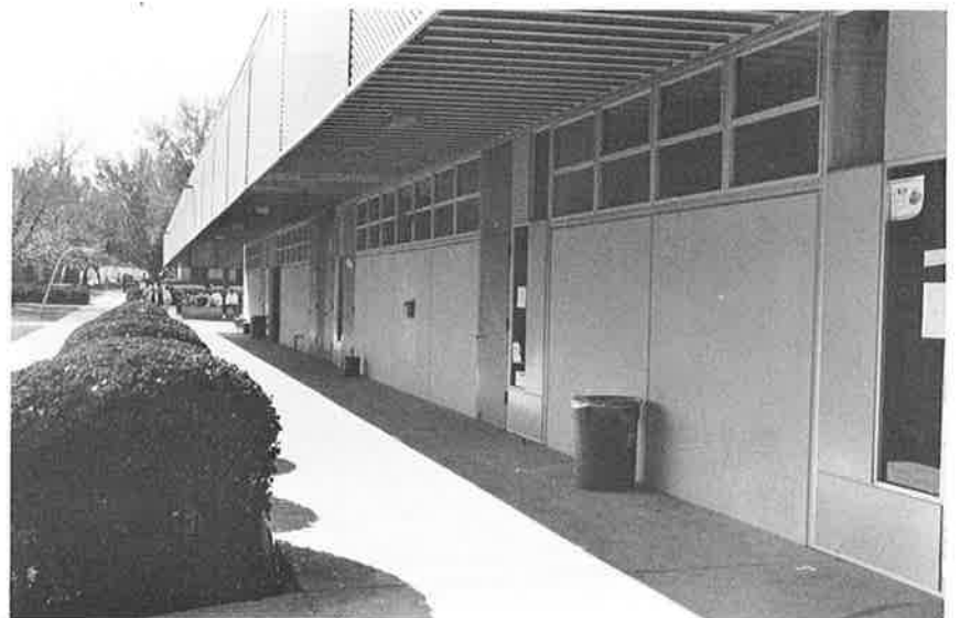
Standardized Outdoor Corridor Design -- Overhangs with expanded metal fascia are effective in providing summer shade, but exterior doors facing into the weather can waste energy.
